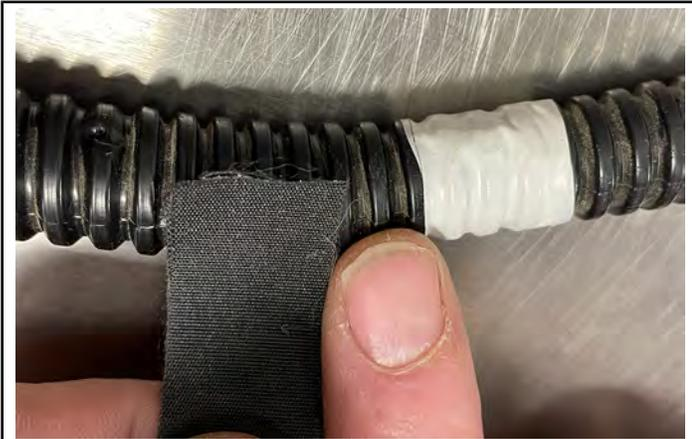
4. Wrap the tape, overlapping each wrap about 50%, until you reach the bottom opening of the conduit.
