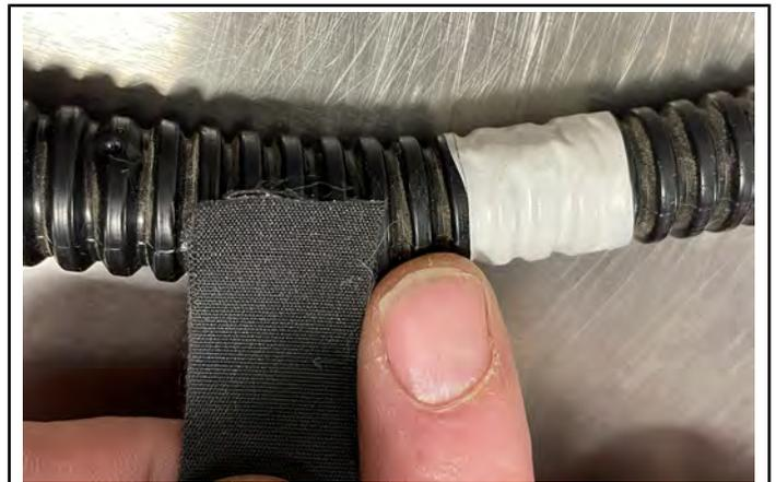
4. Wrap the tape, overlapping each wrap about 50%, until you reach the bottom opening of the conduit.
